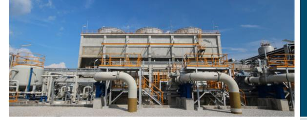
For example, a power plant in Mexico uses grey water (wastewater from sinks and showers generated from households or office buildings) in its cooling tower in an effort to reduce the plant's freshwater use. But grey water can carry high concentrations of calcium, sulfate and chloride, which contribute to scaling and performance issues. Our sales engineers conducted studies to determine optimal cycles of chemical concentration in the cooling tower to minimize water use and avoid scaling.
